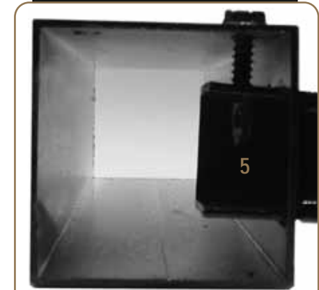
View looking inside post
